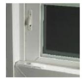
Low-profile tilt latches and sash vent stops add beauty and functionality to the double-hung window.
