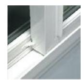
Sash vent stops allow fresh airflow.
